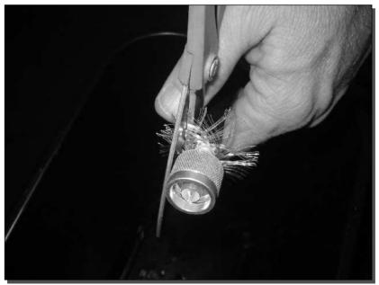
FIGURE 1-23: Trimming the shield with scissors.
